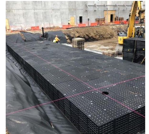
Example subsurface storage detention system
